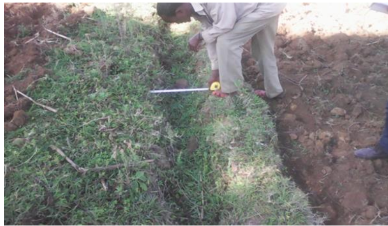
Fig 10: Soil bund after one years of construction
