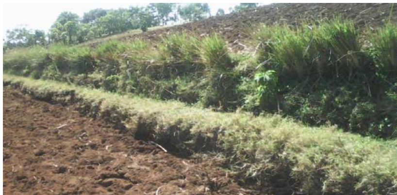
Fig 11: Soil bund stabilized with grass
