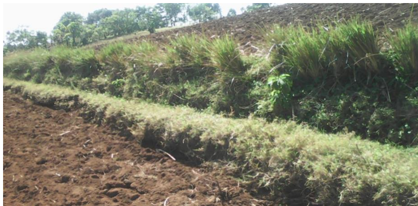
Fig 11: Soil bund stabilized with grass
